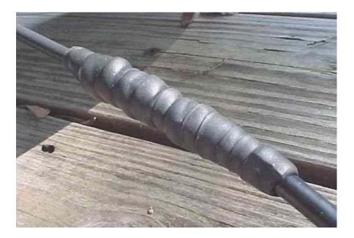
This picture shows : The last wrap again comes straight back over the previous wrap without a diagonal. The seal is slightly sticky and should be molded now by hand to remove any gaps and to ensure that all the wraps are blending together. At some point the wraps will almost fuse together and the material may have to be cut away from the cable.
