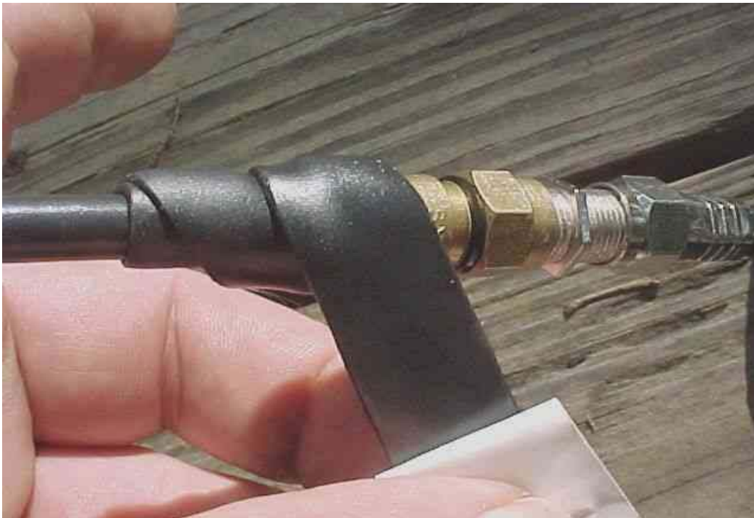
This picture show: Note that the first wrap comes back on itself exactly and the second wrap starts the diagonal wrap. Wrap from the coax cover toward the fitting with one half overlap with each winding.
